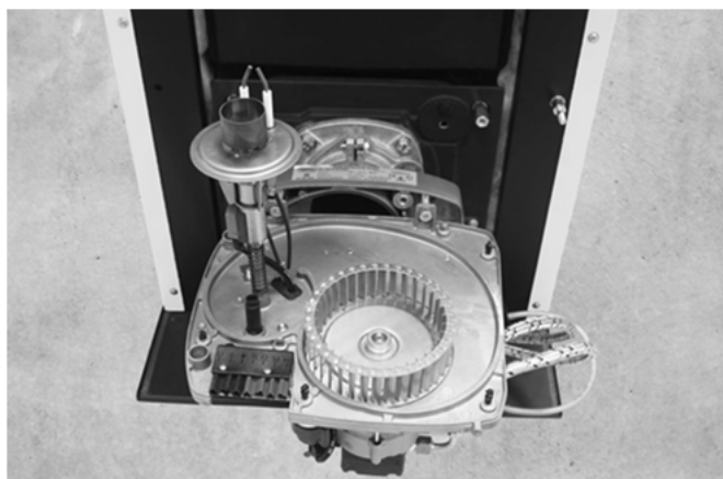
Abb. 33: Brenner in Serviceposition
