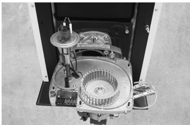
Abb. 32: Brenner in Serviceposition
